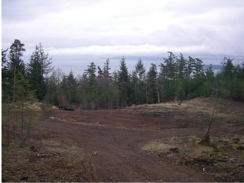
Cleared 2 acre area
